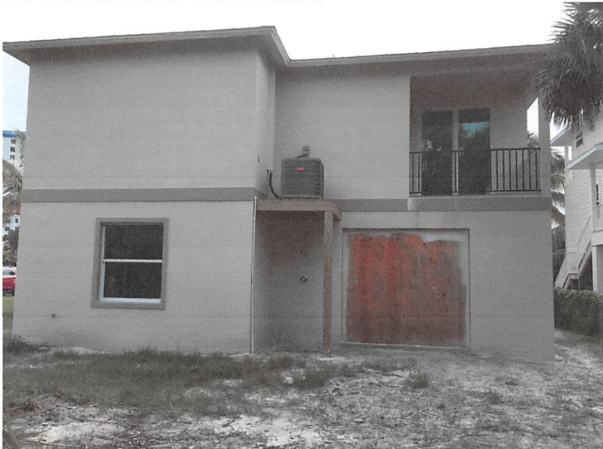
REAR &amp; EQUIPMENT VIEW 1/13/2016
