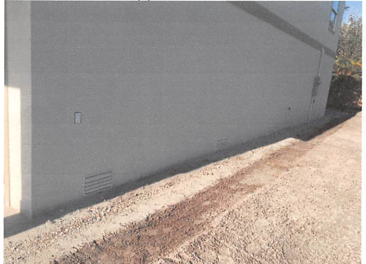
FLOOD VENT VIEW (2) 1/13/2016
