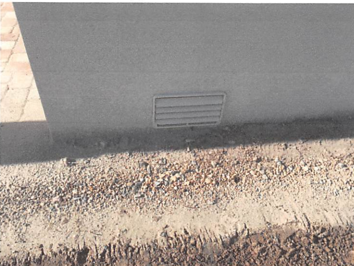
FLOOD VENT VIEW (1) 1/13/2016
