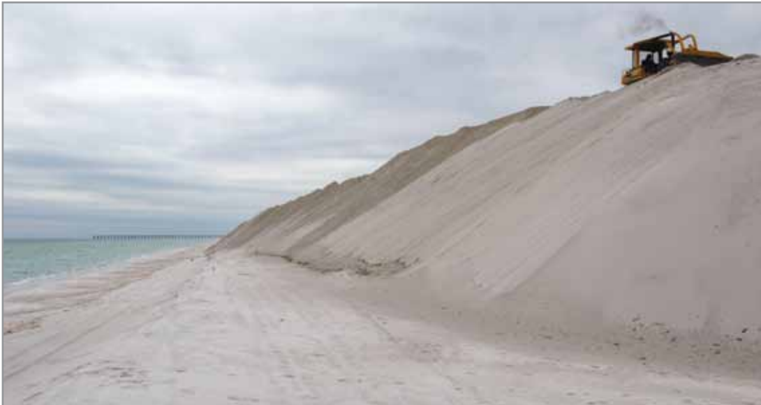
Photo (left): A bulldozer works to repair the sand dune on Pensacola Beach. The dune was destroyed by Hurricane Ivan. FEMA Photo/Mark Wolfe (December 4, 2004, Pensacola Beach, Florida).
