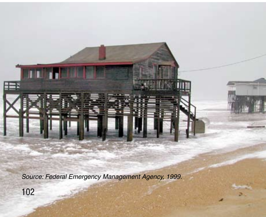
Figure 5.11: Elevation on piles in the V-zone.
