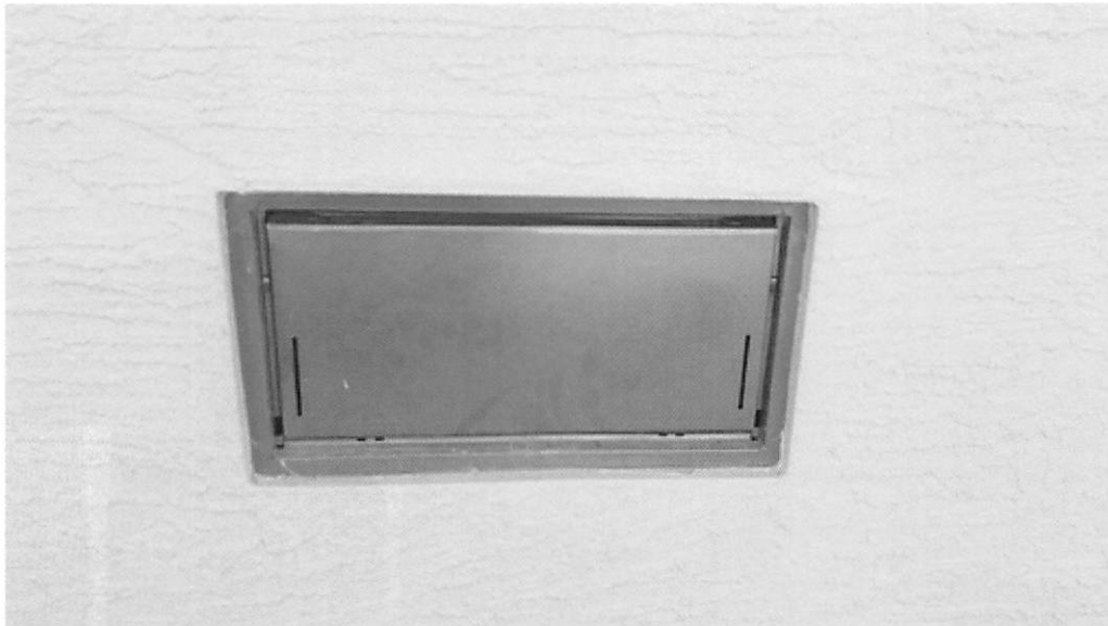
Openings in lower level
